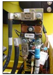
Truck fuse panel assembly
