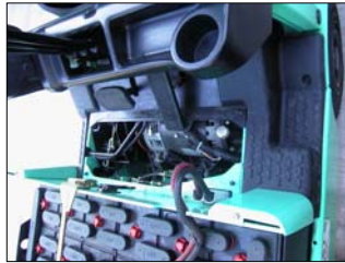
View of motor compartment with drop in floor plate removed.
